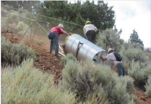
Winch and pulley system used to transport culvert gates and PUF to a closure site at a forty (40) degree slope.
