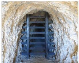
Examples of Culvert Gates installed in Abandoned Mine Hazard adits or shafts that contain loose rock at the portal or collar. Culvert gates effectively increase the life of the closure by preventing collapse of the back or side walls of the AML Hazard. All culverts are installed to the proper length or depth where competent rock exists. The culverts are then secured in place with PUF and backfilled with two feet of native material.
